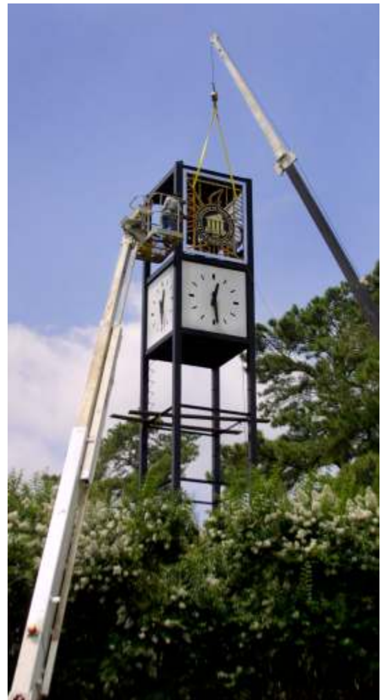
Bell tower during renovation
